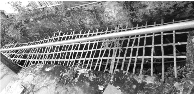
Fig.2: Picture of bamboo mesh in Sangtemla Ward.
