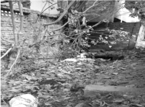
Construction of building over the Drain
