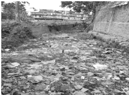
Drain covered by solid waste and sediments
