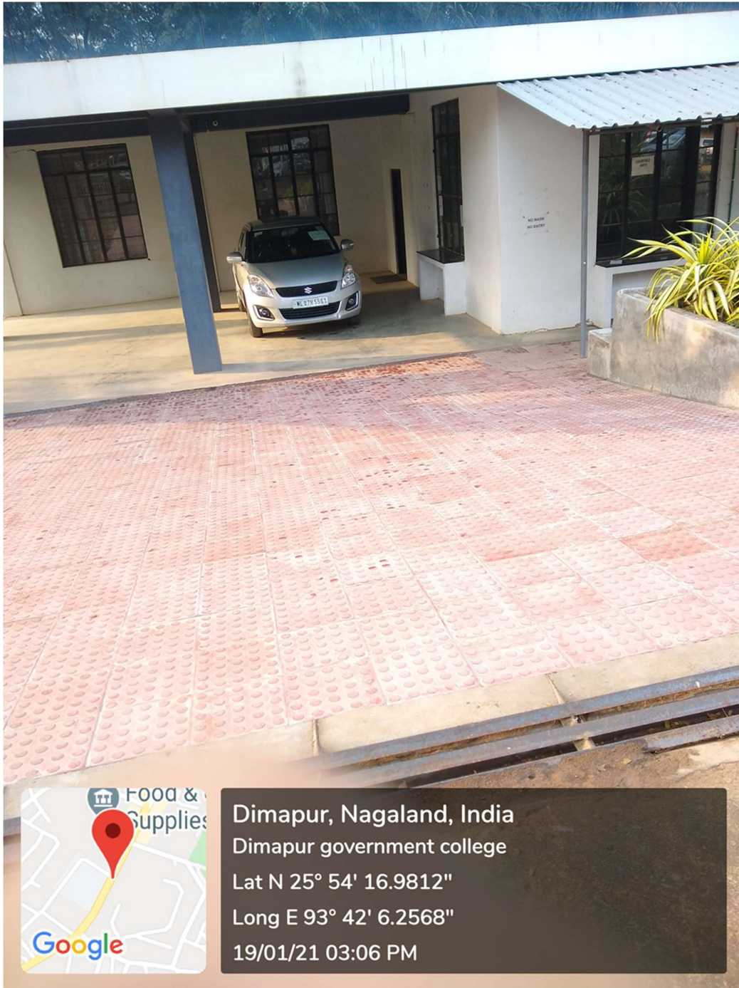
Ramps to the administrative block.
