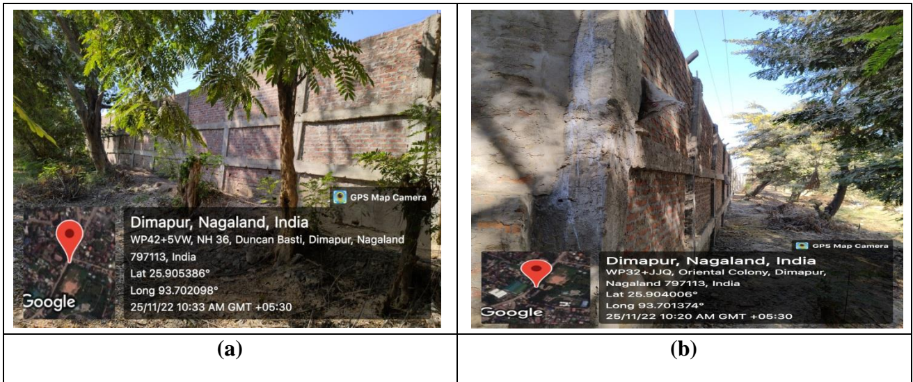
Photograph 13: (a. b) Construction of Wall along the National Highway
