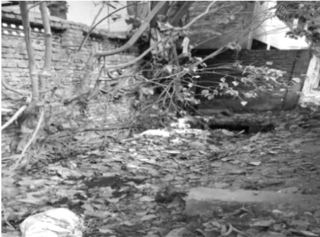
Construction of building over the Drain
